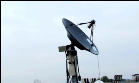
Transmitting antenna reflector 1,8 m, 40dB gain, X-Y positioning, frequency bands VHF/UHF/S (Operational since 2011)
